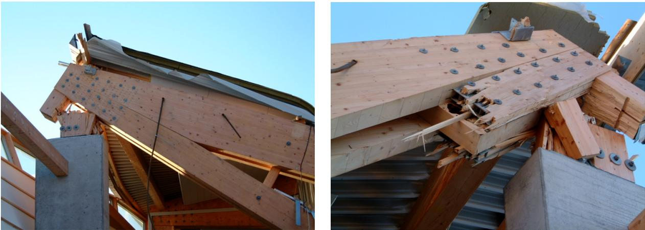
Figure 4.4: Failure of corner connections: (a) due to tension forces (b) due to increased rotation (Munch-Andersen & Dietsch, 2009)
