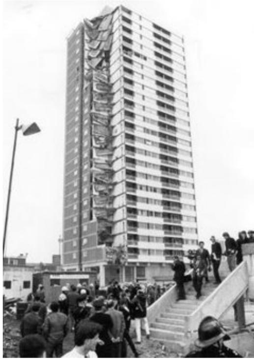
Figure 4.1: Ronan Point progressive collapse
