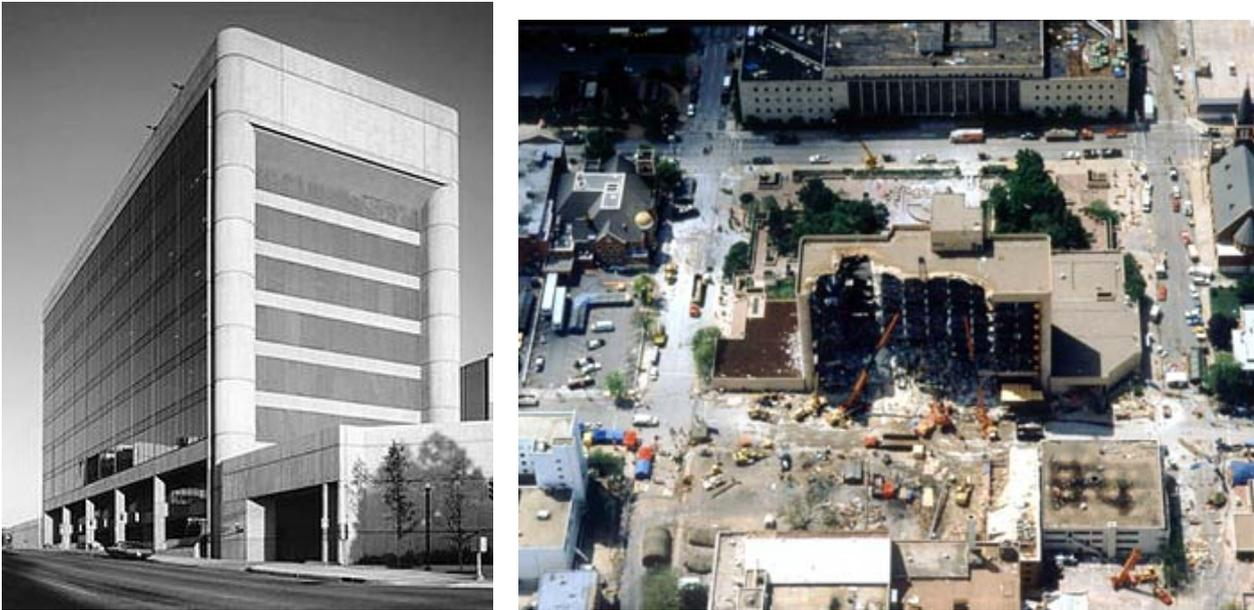
Figure 4.2: Murrah building: (a) intact structure; (b) partial collapse
