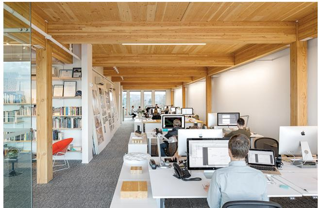
(b) Glulam post-and-beam structure
