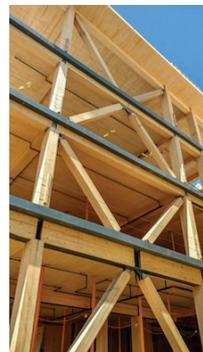
(b) Braced timber frames
