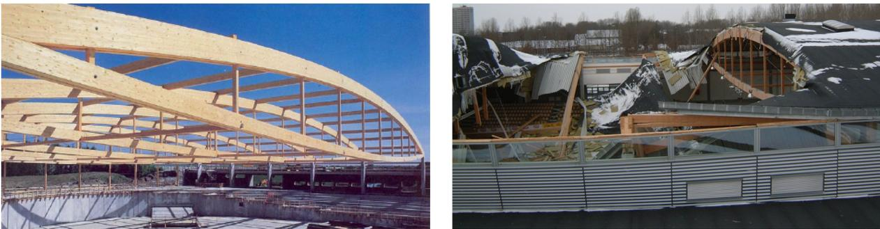
Figure 4.3: Siemens Arena Roof: (a) fish shape truss; (b) failure of two main beams (Munch-Andersen & Dietsch, 2009)
